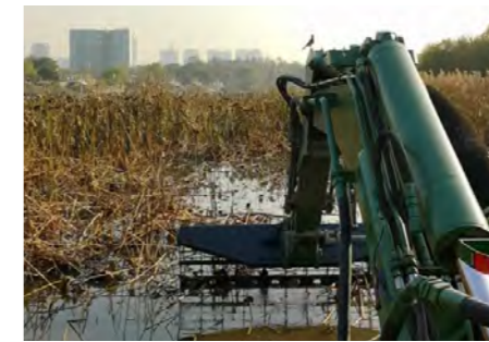
Clearing vegetation and debris by raking
