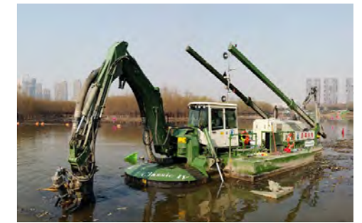
Removing sludge by suction dredging
