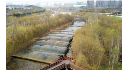
Dewatering with geotextile tubes
