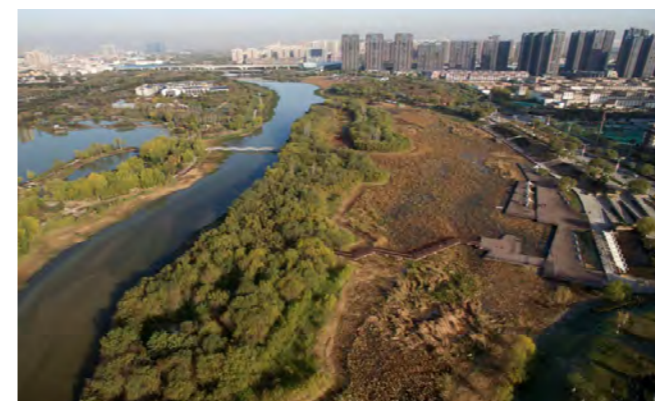
BEFORE restoration Pollution, excessive vegetation and siltation, deteriorating aquatic environment, high risk for floods
