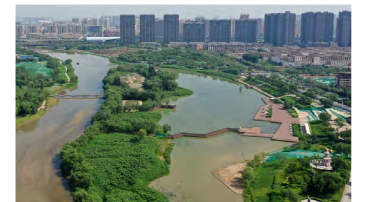
AFTER restoration Cleaner and healthier environment and recovering ecosystems, more enjoyable urban area for locals and tourists, lower risk of floods
