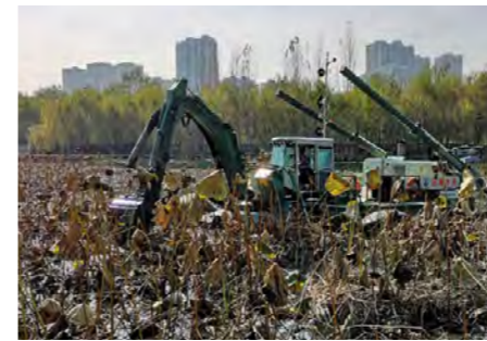
Removing waste and siltation by excavating
